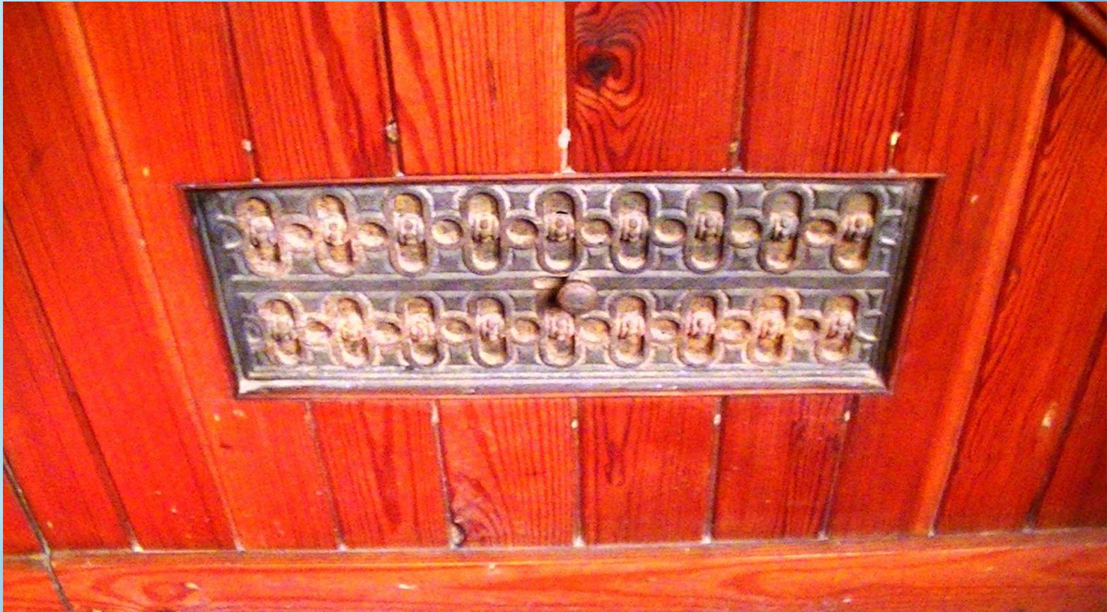
**Looks like a ventilator on the side of the pulpit but it's actually connected by a wooden duct to a heating chamber below the church. It's unclear what sort of fire they used because the chamber is partially bricked up. It would seem to have been pretty basic though - just a big fire with the heat rising by convection up through the church. Apparently it was never a success because it channelled up smoke as well as heat!**
