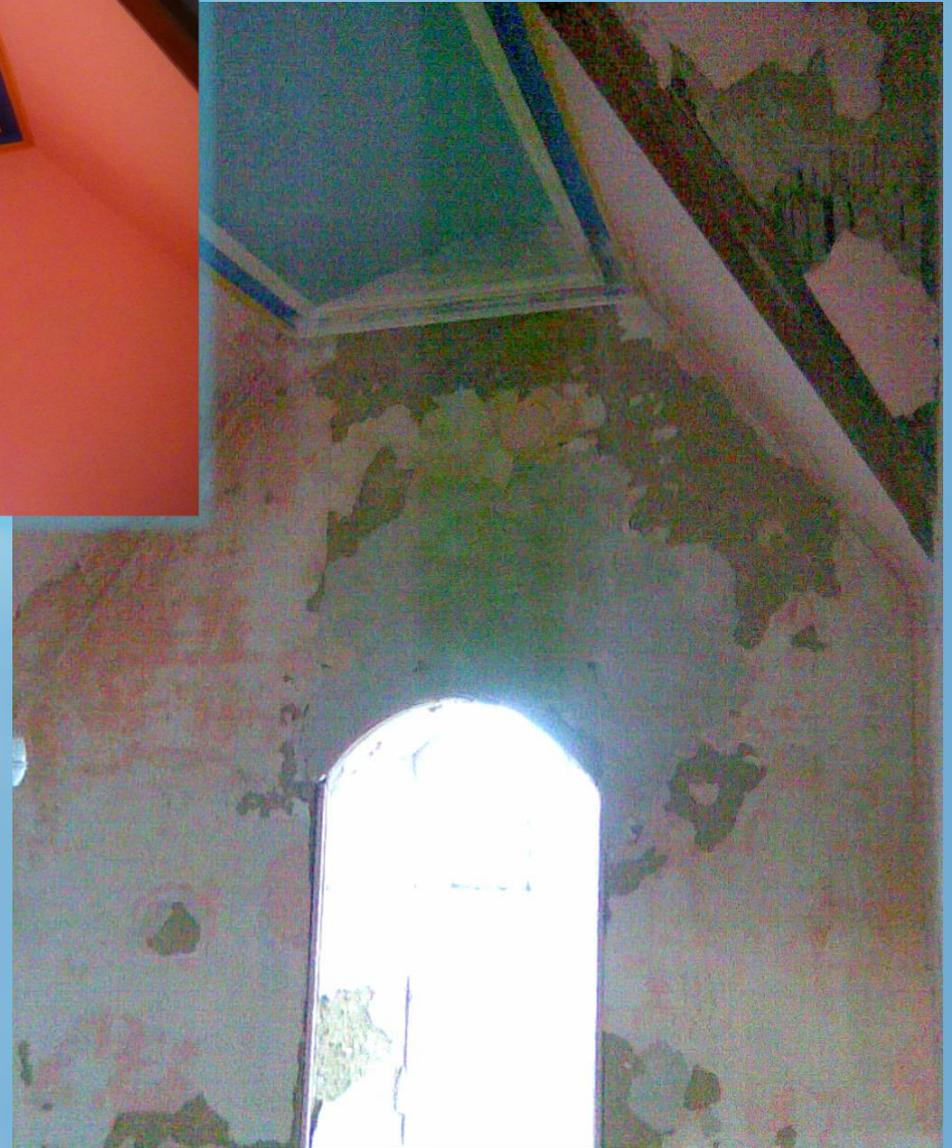
**Upstairs was completely re-lined and the ceiling and cornices were re-plastered as needed. In total we went through 37 sheets of plasterboard!**
