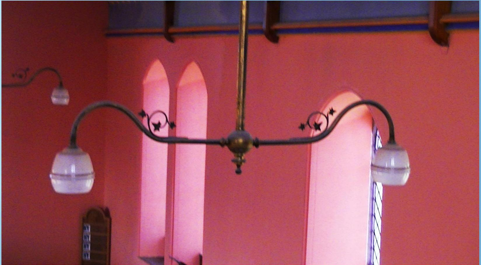
**The brass light fittings were in fact the original carriers for the paraffin lamps before they were wired for electricity. At the top of each light fitting you can still see the pulleys that were used to raise and lower the lamps for lighting. The ropes and pulley system are still there up above the church ceiling - they ran down to the back of the balcony.**
