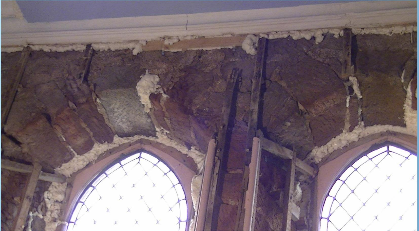
**The upstairs windows were falling out (during the winter of 2013-14 they had to be propped up inside with a pole tied to the end of a pew!) They were fixed back to the stone with metal straps then sealed off with expanded foam inside and silicone sealer outside.**
