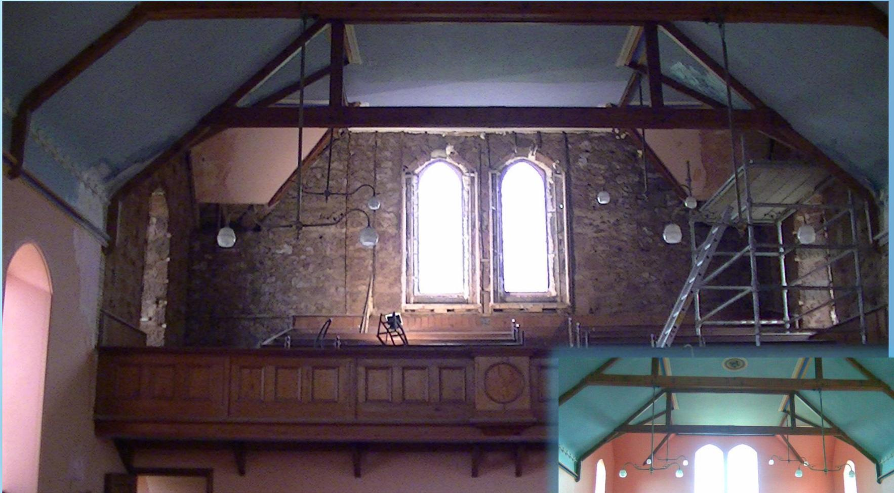
**The whole of the upstairs and the stairwell had to be gutted back to the stonework before putting up new posts and plasterboard.**
